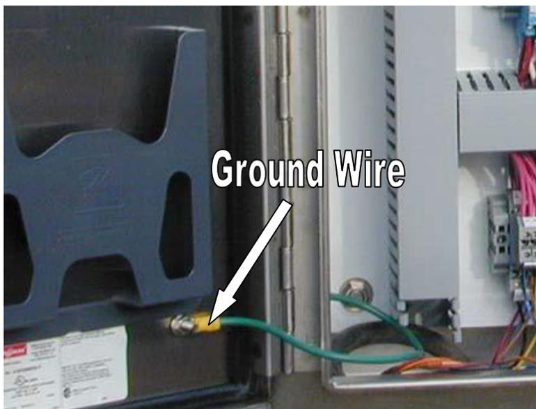
The ground wire provides protection against unequal potential between panel components and the surface on which a maintenance technician may stand while working in the control panel. While the voltage at this connection point may rise above zero volts-to-earth-ground under fault conditions, the entire system will also rise at the same rate to the same voltage. This helps minimize any circulating currents between components from lightning or power surges.
