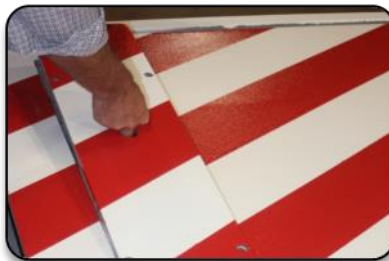
Figure 35, 36, & 37 – Removing the Access Panels
