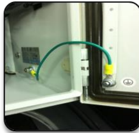
Figure 4 – BCP Ground Wire
