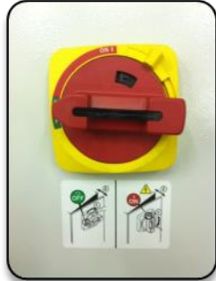
Figure 1 – Main Disconnect
