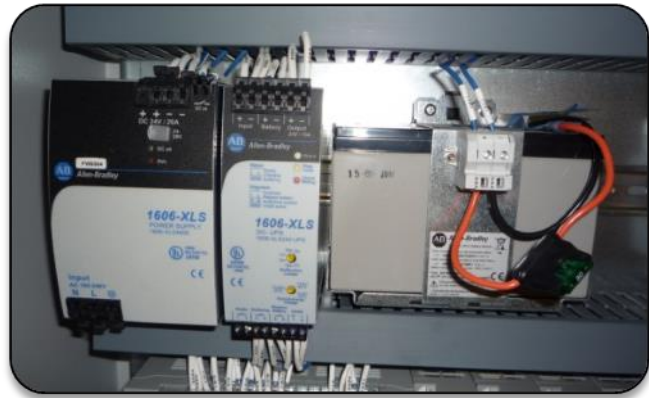
Figure 23 – 24VDC Power Supply & Optional BBU
