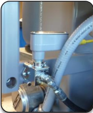
Figure 32 – Pressure Switch
