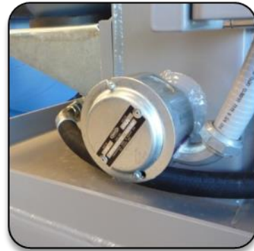
Figure 34 – Hydraulic Heater
