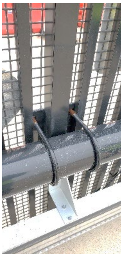
Figure A-4. Attachment via U-Bolts
