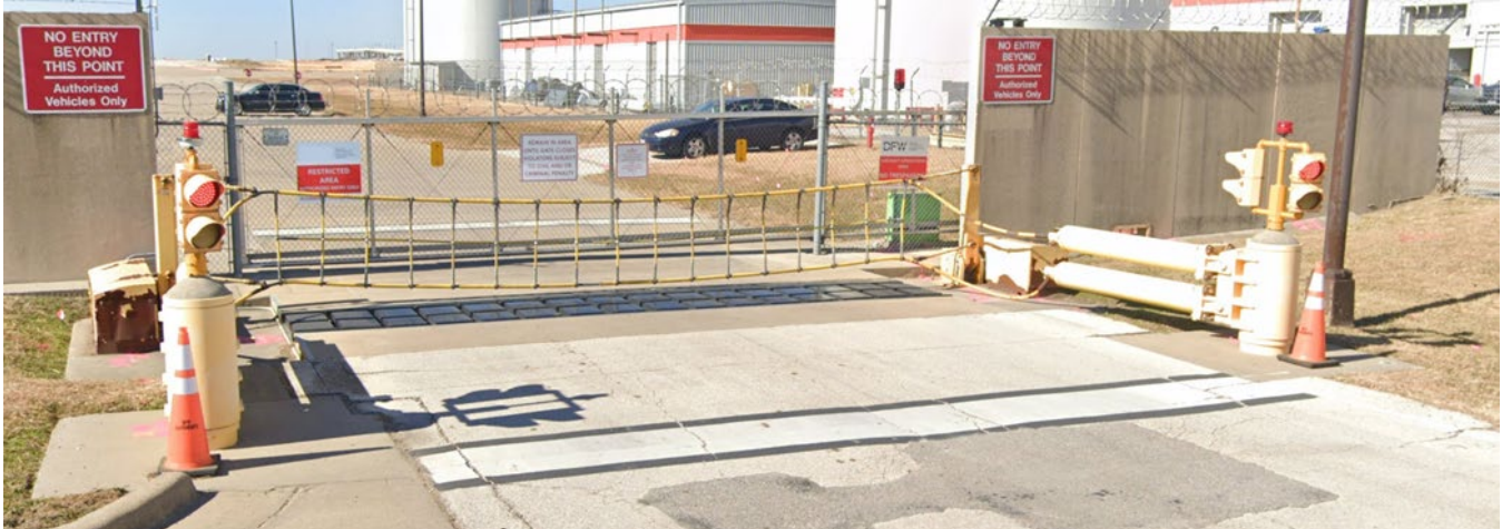
Figure 3-7. Net Barrier at a CAT X Airport
