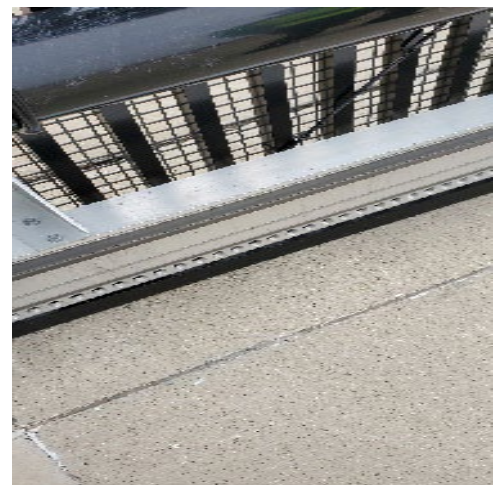
Figure A-6. Anti-Climb Mesh
